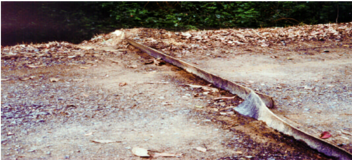
Figure 2 Water disbursement with rubber belting
