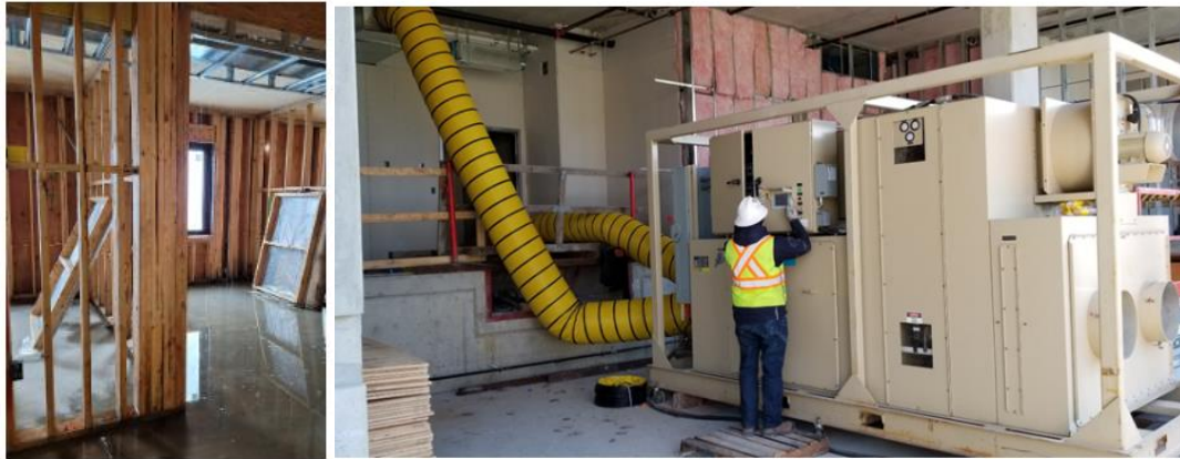
Figure 19: Desiccant drying on construction site.
