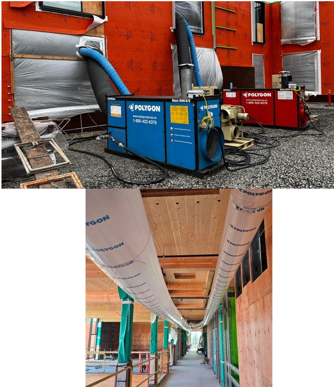
Figure 10: Example of drying process on construction site focused on reducing moisture content using desiccant drying (top) and tunnel fan drying (bottom) [51].
