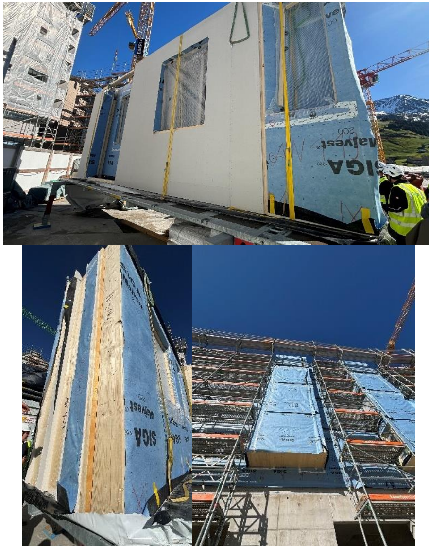
Figure 8: Prefabricated building sections arriving at site protected for any weather change and moisture exposure, Switzerland.
