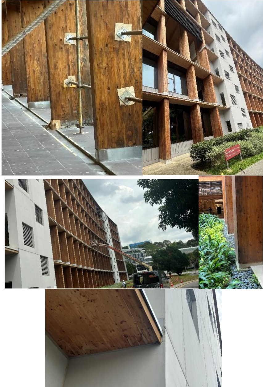
Figure 18: Sections of mass timber building exposed to outdoor environment and maintenance in progress addressing various moisture issues.
