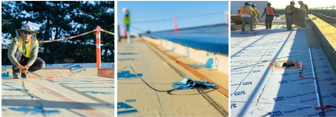
Figure 15: Leak detection systems applied on outer surface of roofing.
