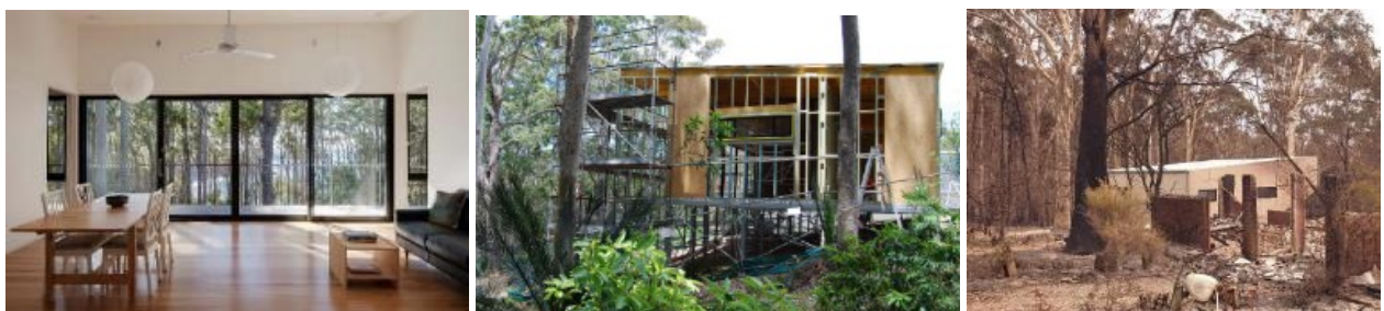
The Rosedale Beach House was designed by Thomas Caddaye Architects to be compliant with AS 3959 Flaming Zone requirements. When a bushfire destroyed or severely damaged 18 nearby homes, this one resisted, with very minor repairs (some window gaskets, an outside plastic light over the door and the external PVC plumbing pipes). There was no hint of smoke indoors. Construction costs (in 2017) increased by about 20-25%, but it was still an affordable house, and looking at the result it seems worth it.
