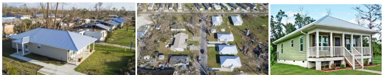
Six Habitat for Humanity houses came through Hurricane Michael essentially unscathed (from: JLC and Strongtie ).
