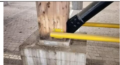
300mm concrete foundation footing
