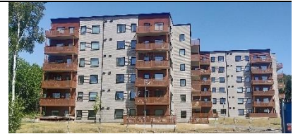
Adjacent completed building showing self-supported CLT balconies.
