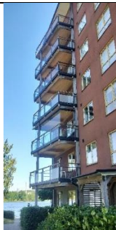
Limnologen site with supported timber balconies and rendered ETICS façade.
