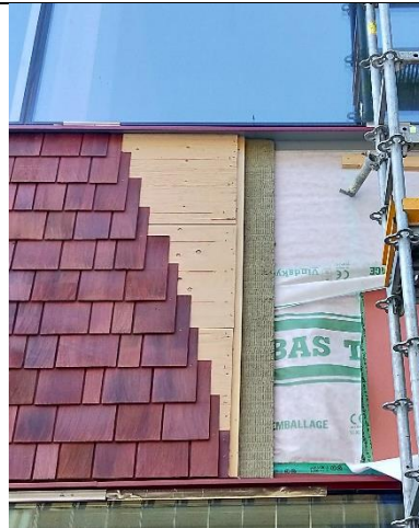
Build-up of wall assembly layers clearly visible
