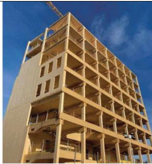
Completion of the timber erection (Overton et al., 2023).
