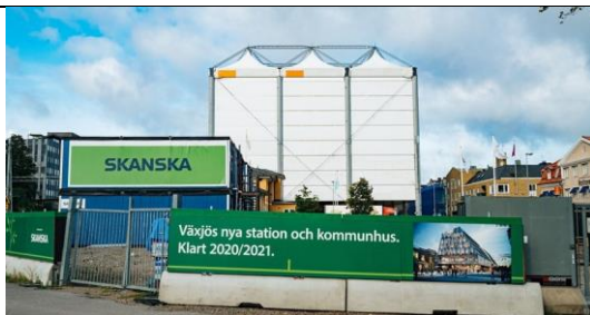
Site built under a full tent for the duration of construction (Skanska, 2024)
