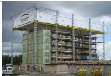
Tenting strategy for stormwater protection (Serrano, 2009).
