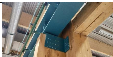
Structure of factory comprises of glulam columns .
