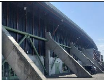
Outdoor concrete supports.
