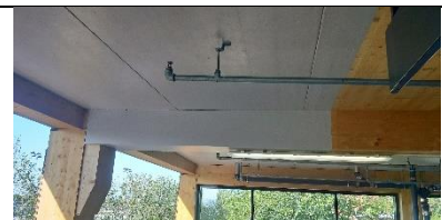
Intumescent coating applied at perimeter
