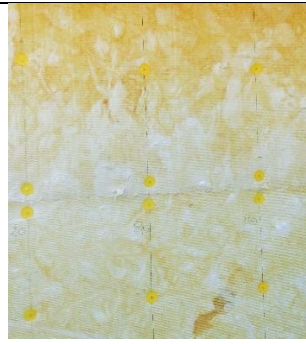
Meticulous installation of semi-rigid insulation panels mechanically fixed to external wall.
