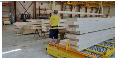
31 m glulam beams maximum length
