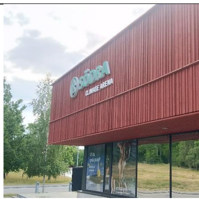
Highly reflective glazing treatment.
