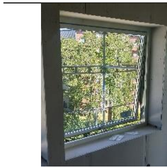
Interior view showing depth of window reveal.
