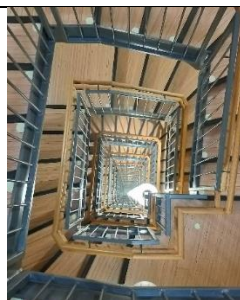
Timber staircase and CLT core.
