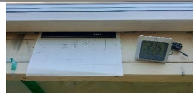
Onsite measuring monitoring of CLT moisture content
