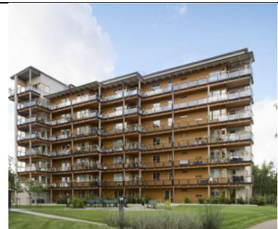
Complete building (Žegarac Leskovicar and Premrov, 2021).
