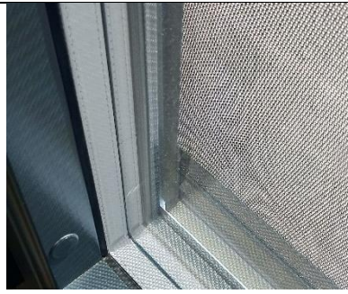
Triple glazed window with operable external fabric elements.
