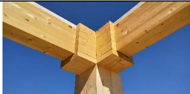
Glulam beams showing membrane applied to horizontal end grains and surface wax treatments
