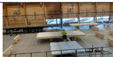
Membrane is manually adhered before shipping.
