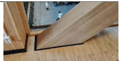
Large glulam pillars are visible and make a design statement.
