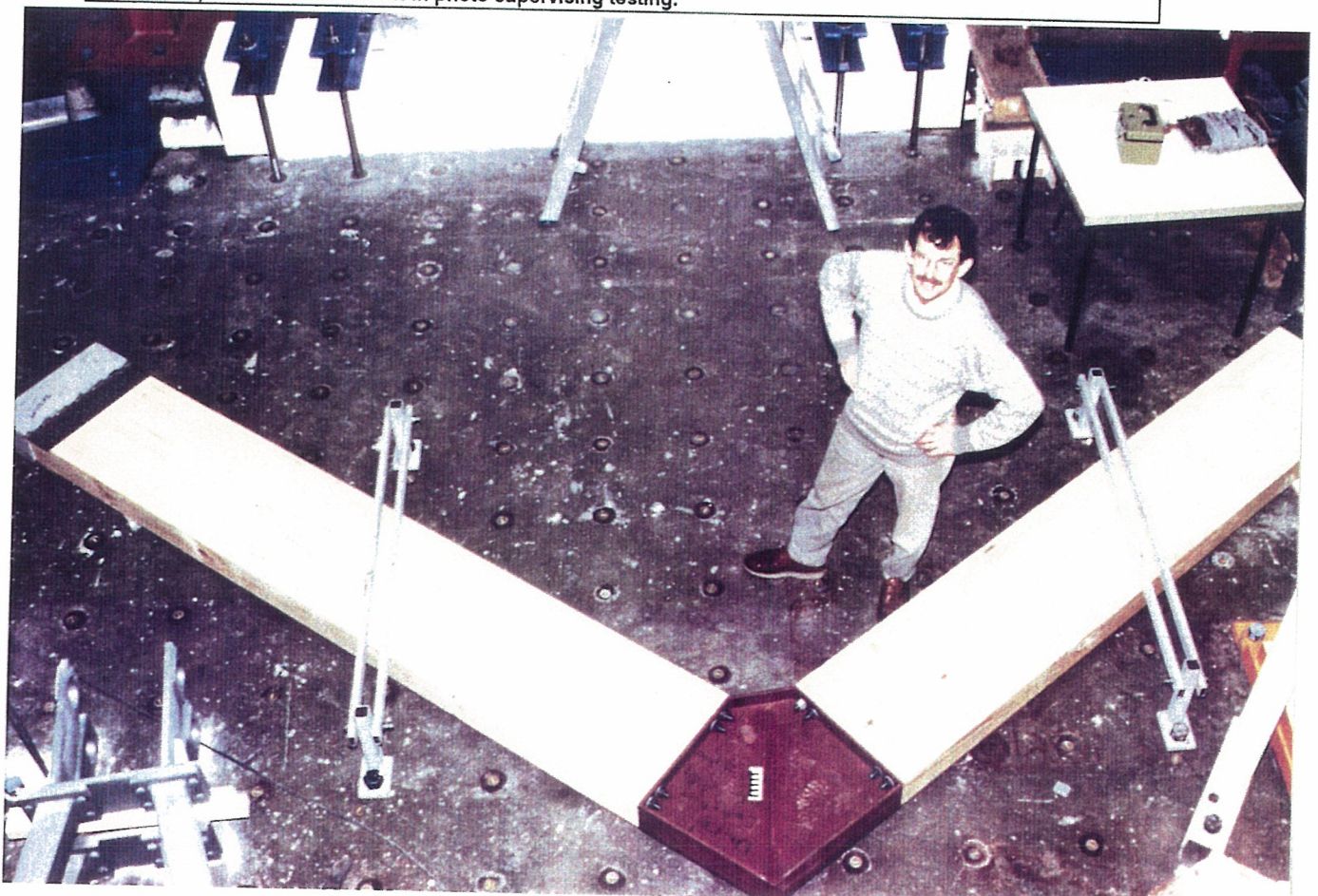
Photograph 2.12 - Steel portal haunch using epoxy injected rods (note: connection is patented by Hunter Laminates) Dr Buchanan shown in photo supervising testing.
