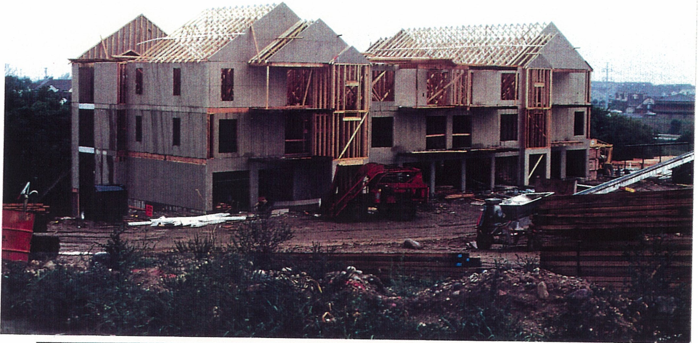
Photograph 5.1 - 3 storey MSTF residential construction near Madison Wisconsin, USA
