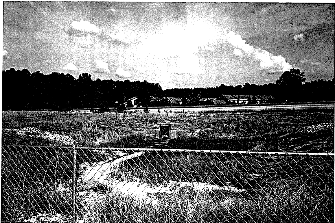
Plate 4.8: Stormwater discharge basin with isolating drain outlet.
