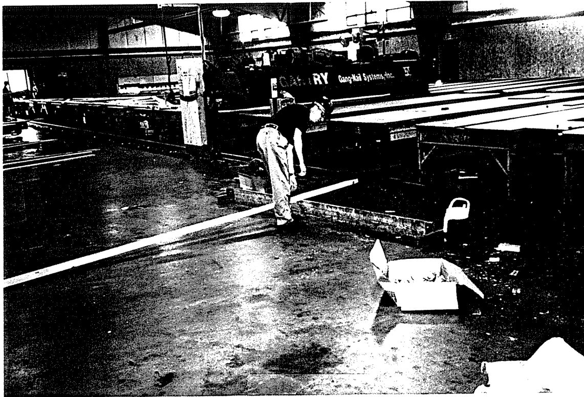
Wood Structures the simplest device (2"x 12" length of timber on edge, with support ends affixed), serves to minimise stooping to the floor to retrieve truss components
