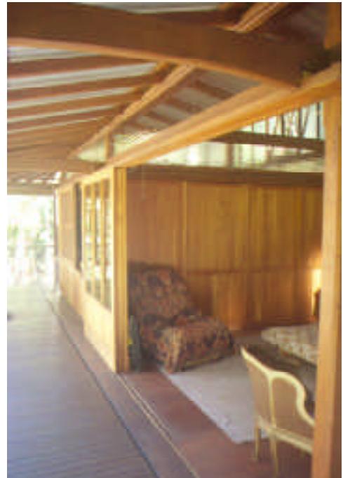
Above: sliding screen doors supported in a floor track and from the main roof beams. Note the detail of the threshold, the recessed track and the flooring that reduces water penetration whilst keeping the floor levels flush.
