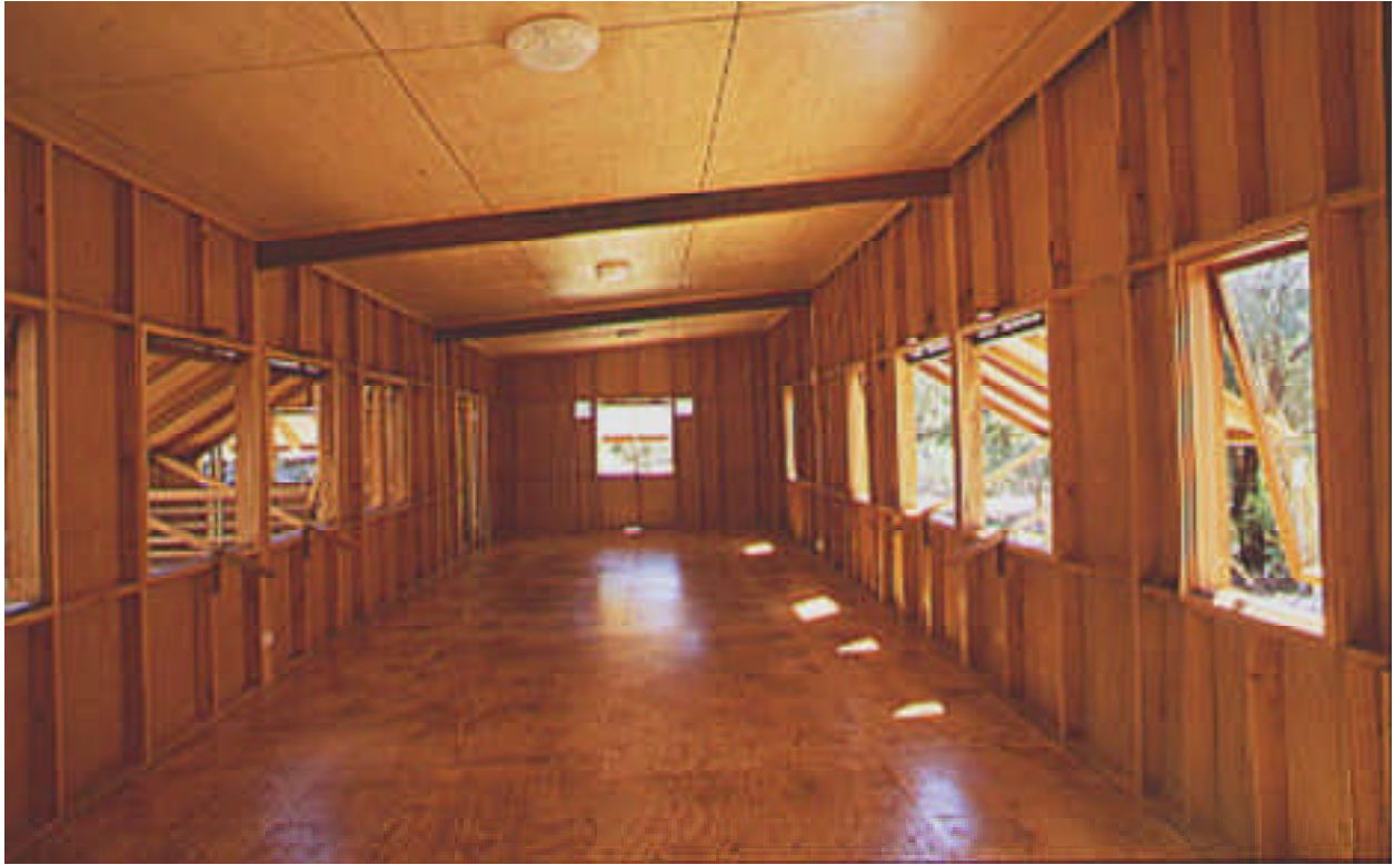
Above: interior stain finishes to the plywood are low cost and durable.
