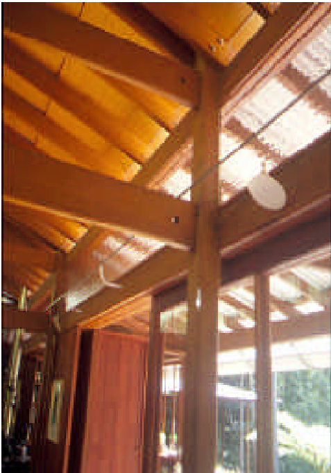
Below: three dimensional interlocking joints for the upper frame triangulate the roof structure.
