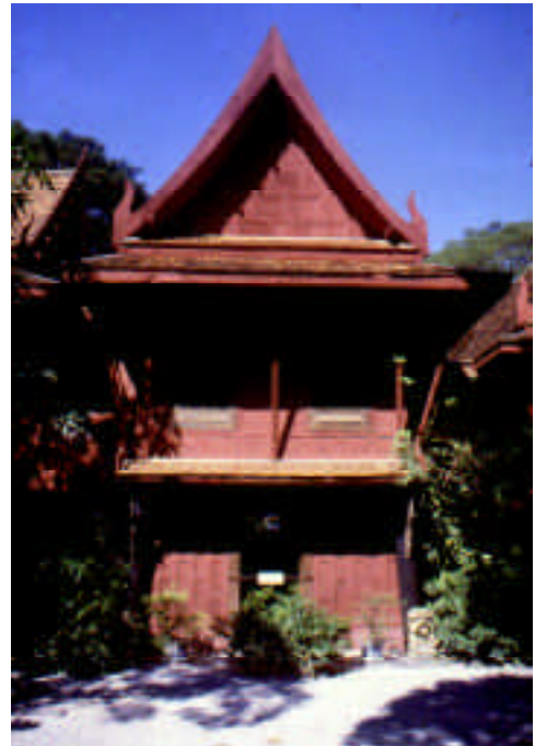
Above: Jack roofs are used to provide shading and protection to the timber single skin construction. These are braced to the floor elements. Traditional ornamentation gives a symbolic and cultural purpose to elements of the building.
