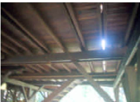
Below: two way bearer system is used to support the floor joists. Additional two way knee bracing is used as a subfloor bracing system.
