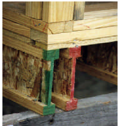
Above: a combination of new engineered products such as I-beams and recycled timber used in the project to reduce the amount of new resources used.
