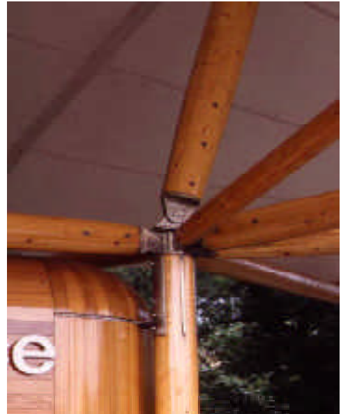
Above: pin joints are used extensively for the tension structure which appears to be braced by the cabin below. Tensegrity principles are used in the design of the structure with an expression of compressive and tensile forces in the design of the members.
