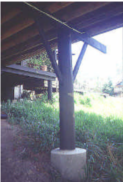
Below: pole frame structure is combined with knee bracing to give stability.
