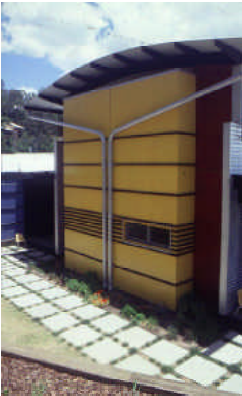
Above: easterly elevation minimises glazing to avoid heat gain. The organisation of the elements is created using Mondrian concepts.
