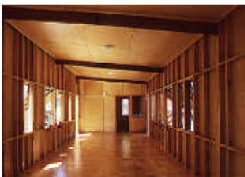
Below: interior space showing the expressed wall, floor and roof diaphragms which brace the structure.
