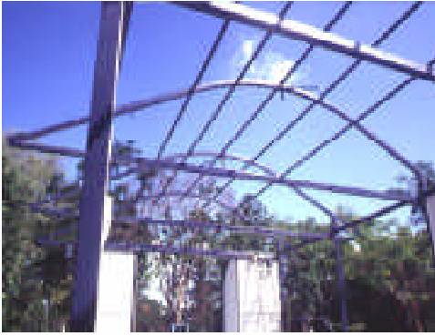
Above: a fabric roof is stretched over the bow string roof truss.
