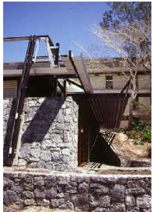
Above: the structural system is based on a concept of cantilever upon cantilever.
