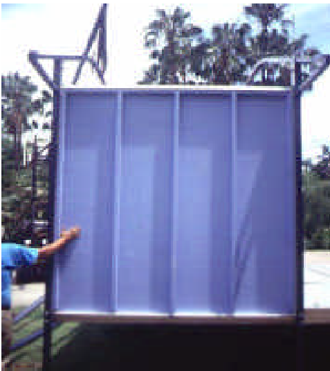
Below: a typical bay of structure showing the 'P' columns that brace the frame.
