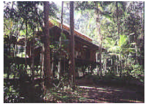
Above: the wrap-around verandah is a feature adopted from the Queenslander house to protect the lightweight skin and allow the building to be opened in all weather conditions.
