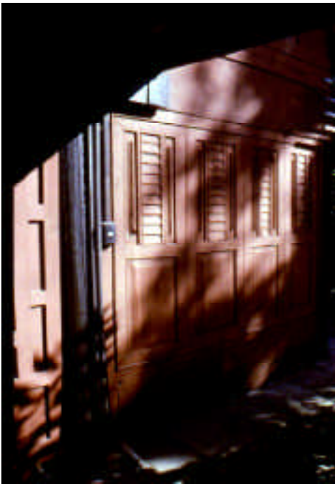
Above: single skin panels are prefabricated and set in plane with the pole frame structure.
