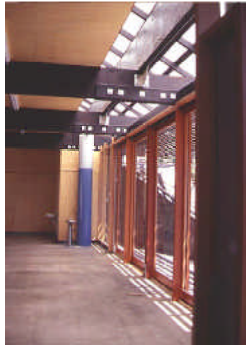
Above: Red Cedar horizontal sliding doors use structural glazing to brace the door panels. The detailing of the LVL timber structure relies on flitch plates to make the connections and stiffen the beams. Note the hanging beam to maintain the headroom and cantilevered shading systems.
