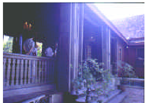
Below: details of the windows and wall framework. The full height bifold door system can open the living area maximising ventilation required for thermal comfort in the hot humid tropics
