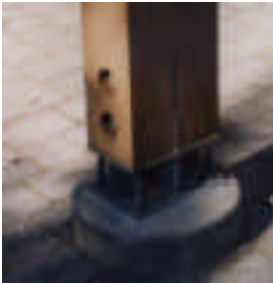
Above: details of the slot mortice system used to hide the steel plate connection system.
