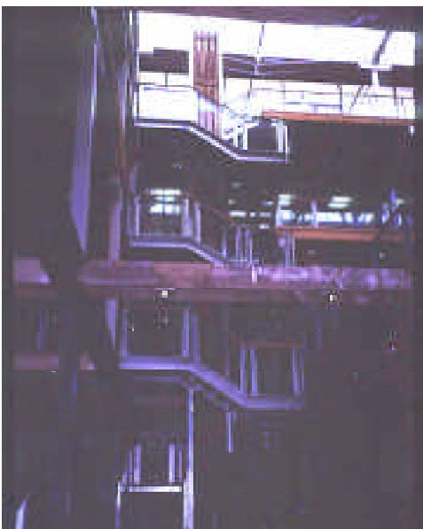
Below: atrium spaces are created in the existing volume and new staircases introduced to improve circulation between levels.
