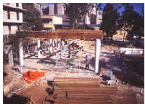
Below: columns provide cantilevered bracing for the main structure, transferring windloads to the foundations.
