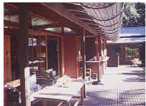
Above: detailing of the roof includes a large gutter to collect rainwater for recycling and is developed as a design feature.
