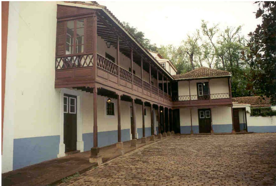
FIGURE C6. This 100 year old balcony on a house near the village of Terror is constructed with P. canariensis heartwood.
