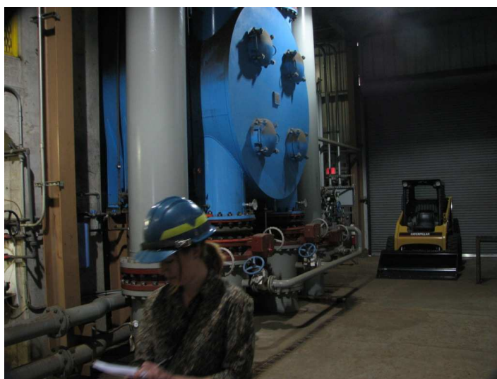
The condenser for the turbine which collapses the residual steam back in to condensate for re-use.
