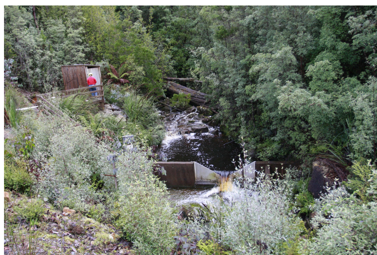
Figure 5. 120 degree v-notch weir and instrument shed at Warra Creek, showing typical riparian vegetation
