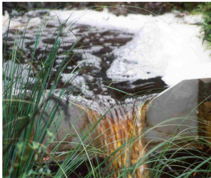
Figure 1. Warra Creek – example of a 120° V-notch Weir used to gauge streamflow in a forest
