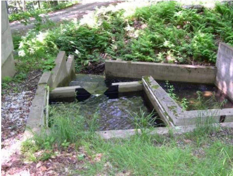
Figure 31. Example of weir designed to accurately measure low and high flows at Hubbard Brook
