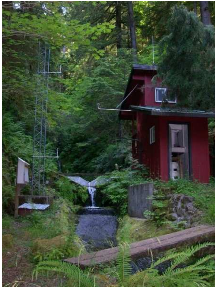
Figure 23. Example of weir and instrument shelter at HJ Andrews – summer weir is in place
