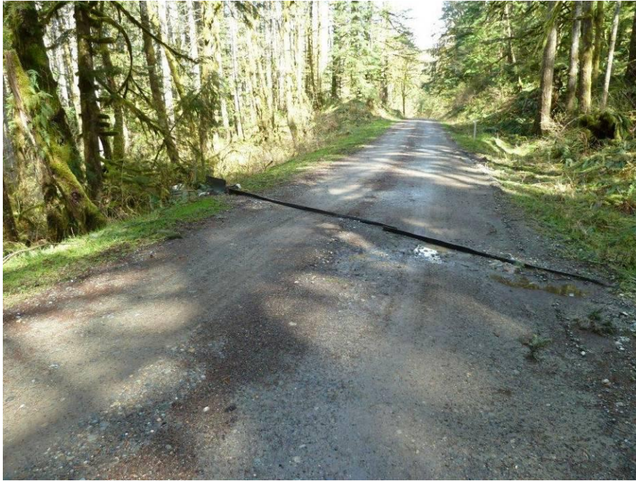
Figure 40. Roads within the Cedar River watershed are well gravelled and drained. Pictured is a temporary rubber flap drainage device being used in a sediment monitoring project
