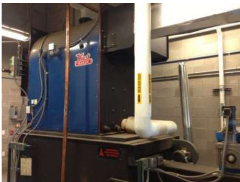
Figure 11. Biomass boiler at Colorado State University, Fort Collins
