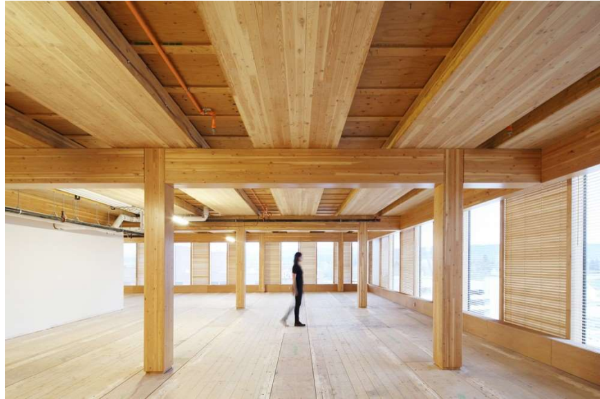
Figure. 4. Provision for ceiling services in WIDC building (Source: Michael Green, http://mg-architecture.ca/work/wood-innovation-design-center/ )
