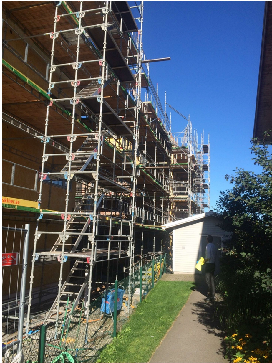
Figure. 10. Panelised construction on 4 storey apartment building
