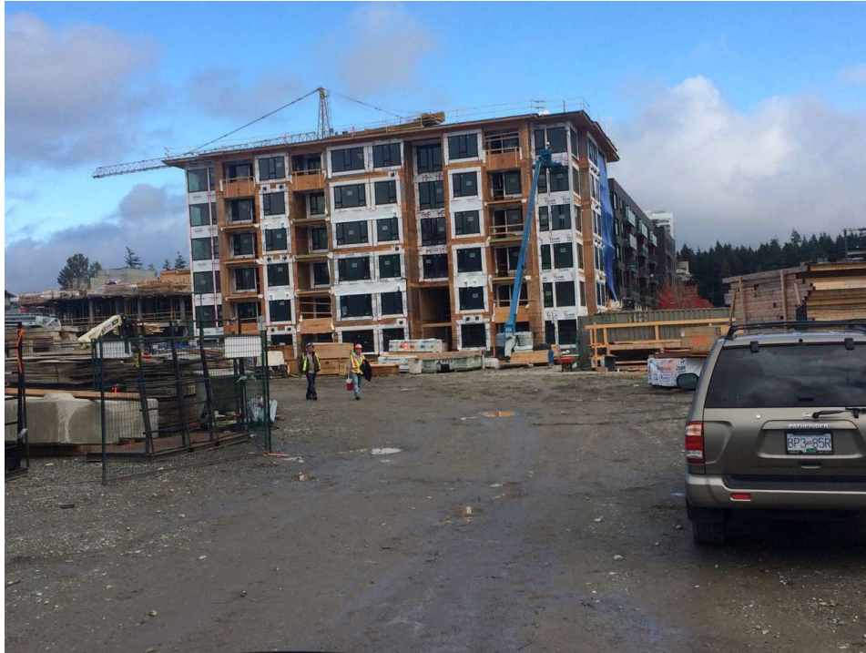
Figure. 1. “Stick built” framed apartment construction in Vancouver
