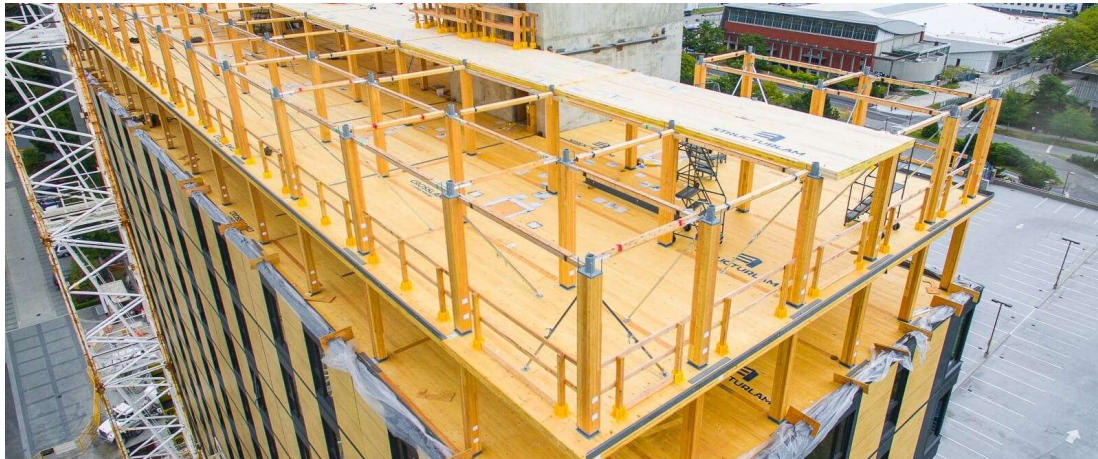
Figure. 7. View of typical floor plate erection on Brock Commons building (Source: http://www.naturallywood.com/emerging-trends/tall-wood/ubc-brock-commons )
