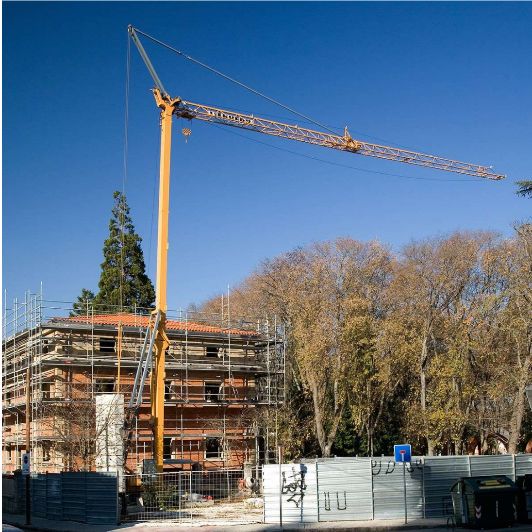
Figure. 18. Liebherr 32H lightweight, fast erection crane (source: https://www.liebherr.com/en/deu/products/construction-machines/tower-cranes/fast-erecting-cranes/h-cranes/details/71141.html )
