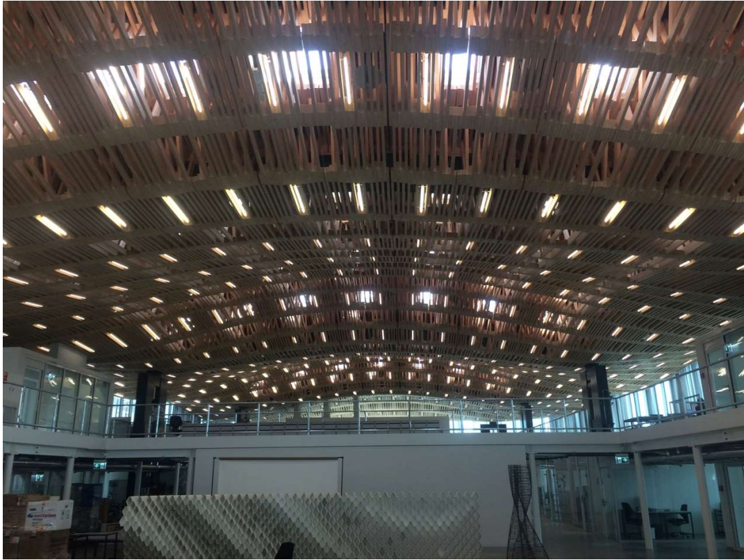
Figure. 16. ETH Zurich, Arch Tech Lab, Trussed roof showing complex geometry
