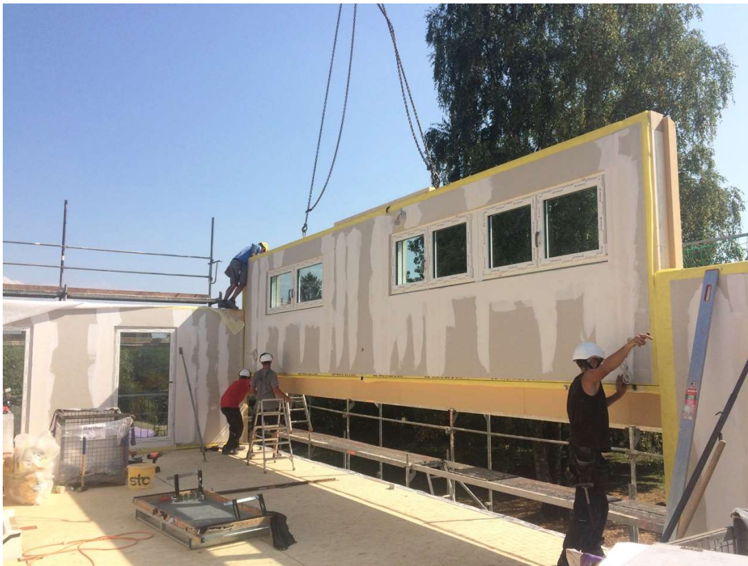
Figure. 14. Closed panels being installed on housing in Germany
