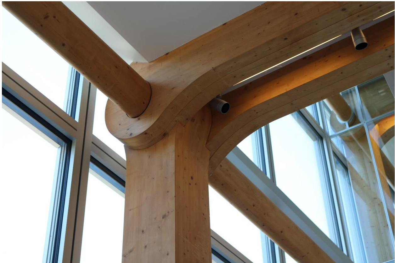
Figure 27. The Junction of the column to beam is entirely timber in construction, there is no steel hardware used. Photo by Author.
