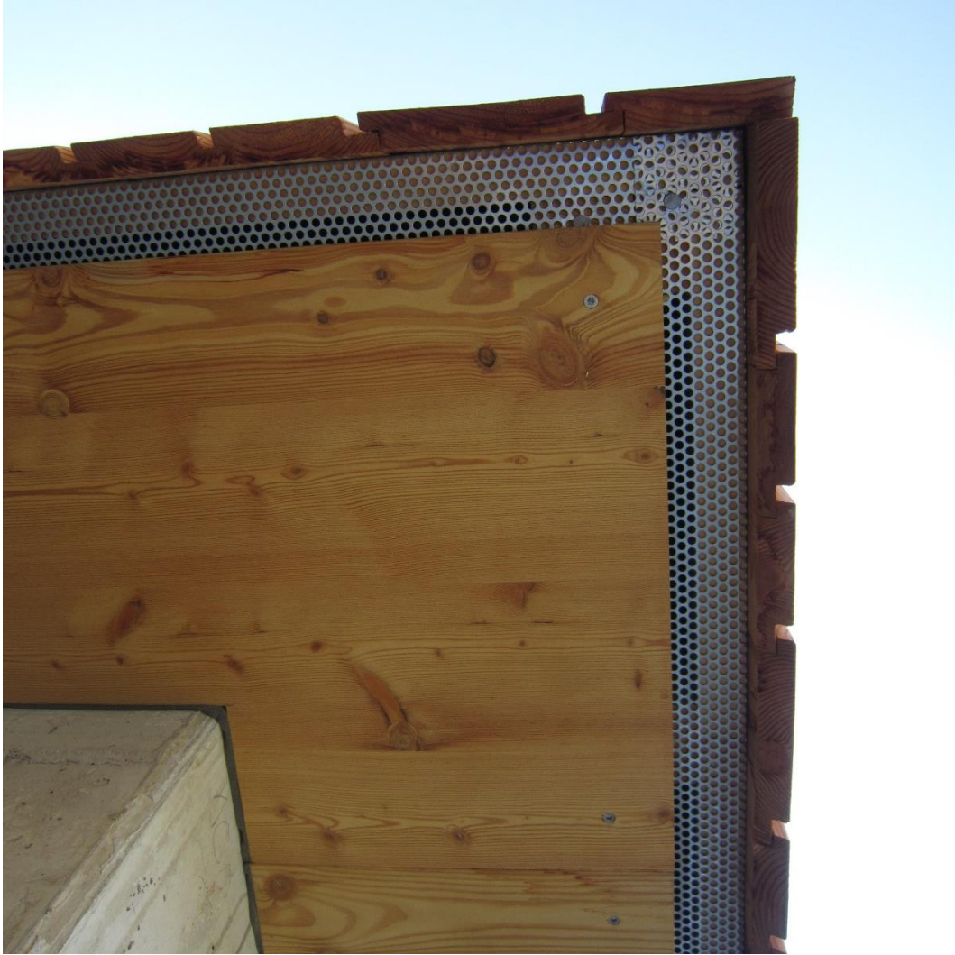
Figure 10. Detail of the floor to cladding. Note the perforated mesh at the base of the ventilated cavity behind the cladding enabling moisture equilibrium on either side of the cladding. Photo by Author.
