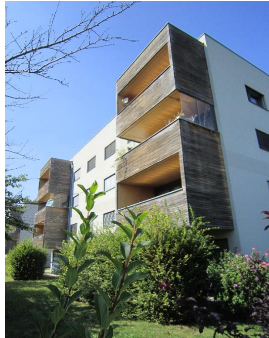
Figure 4: Same building in 2016. Example of weathering of the cladding compared with the CLT exposed in soffits and balcony linings. Photo by author
