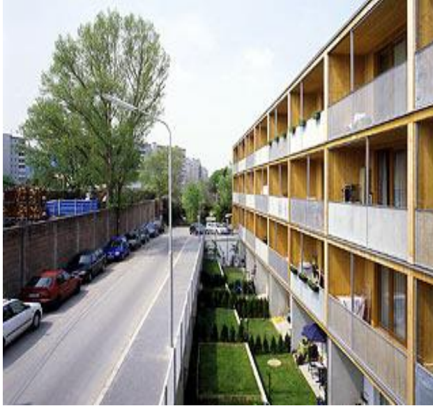
Figure 1 The Spottlgasse Housing project in 2005 A 4 storey building with a concrete structure on ground floor and phot 3 levels of CLT construction above. Photo Pez Hejduck
