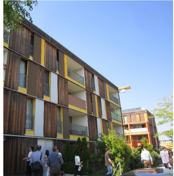
Figure 8. The sSame project in 2016: note the change in timber hue, and influence of the projecting fire protection upon the change in weathering of the timber. Photo by Author.
