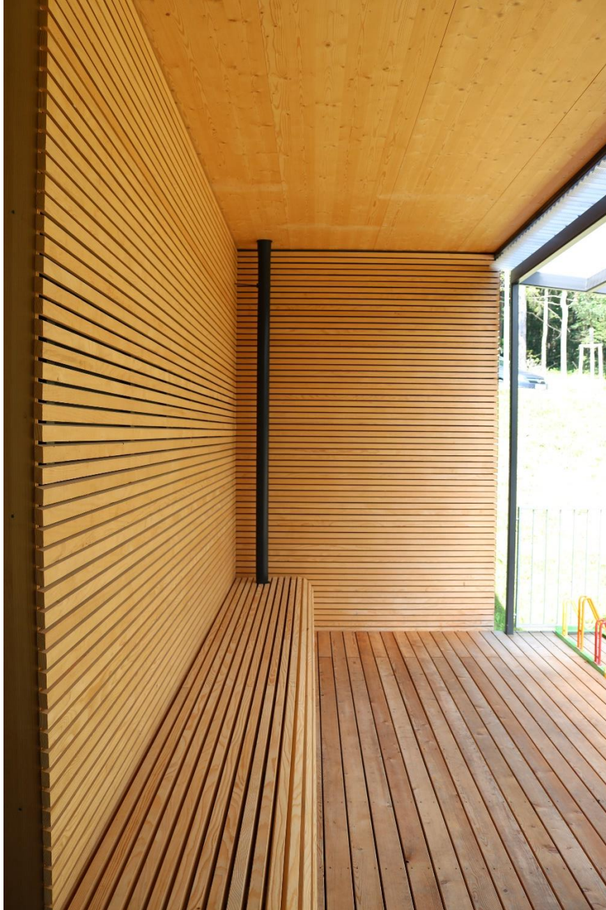
Figure 15. The entry court, with White Fir cladding and a CLT structure. Photo by Author
