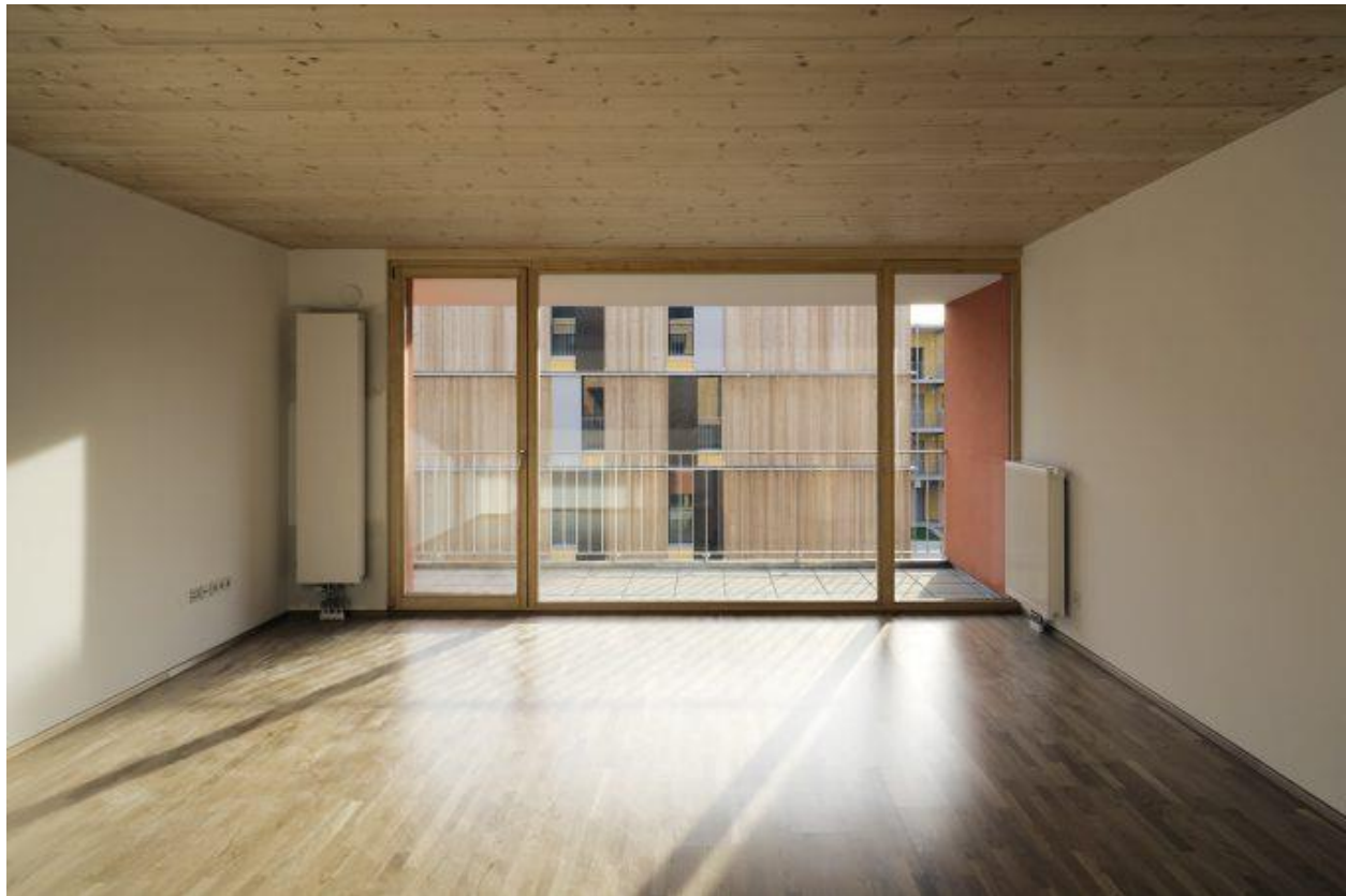
Figure 6. Muhlweg Housing by Kaufman and Kaufman. Note the exposed CLT structural floor in the interior also provides the ceiling for the space, whilst the floor is visibly overlaid strip flooring as it is constructed on top of several insulating layers. Photo by Kaufman and Kaufman
