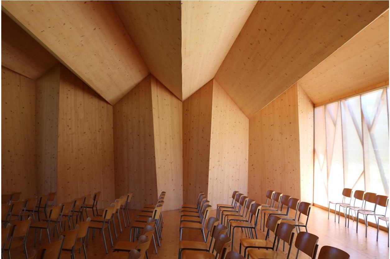
Figure 28. The folded geometry of the timber plate walls provides a unique interior volume combined with a rational, inherent stiffness to the wall and roof planes. Photo by Author.
