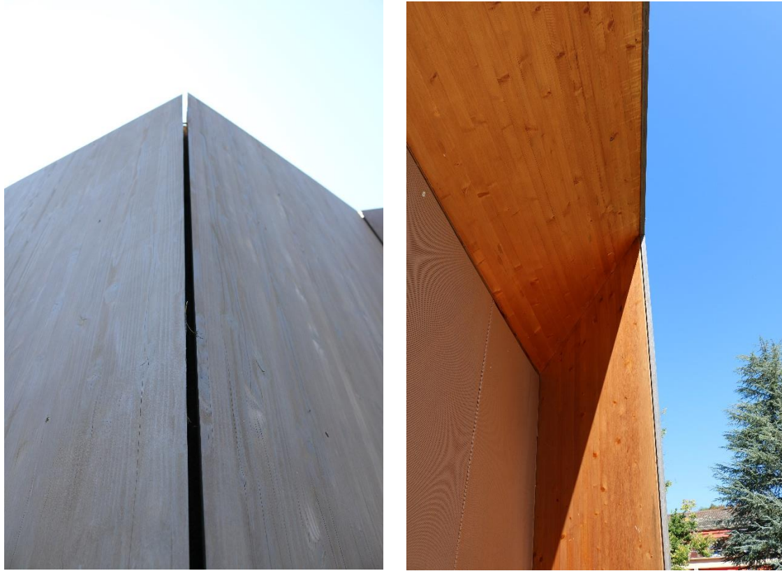
Figure 30. The CNC machining of the panels as can be seen, is very precise, with multi axis mitre joints achieved. Note the ventilation and drainage gap in the exterior ply cladding on left. Photos by Author.
