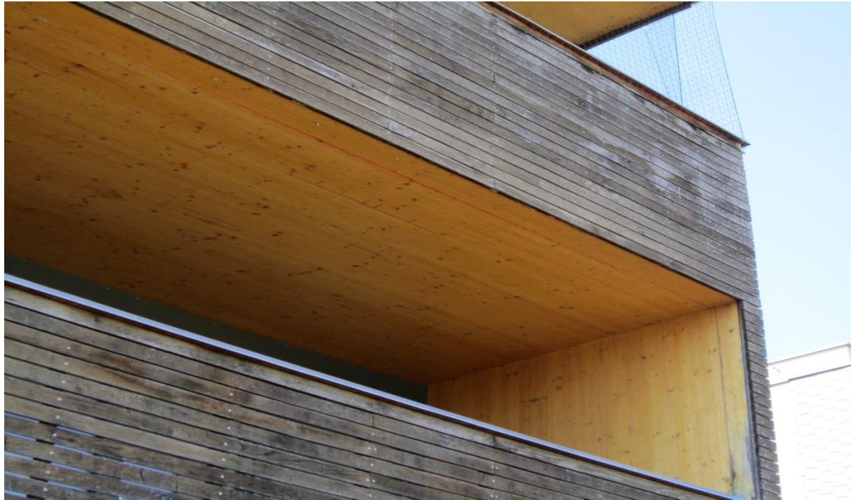
Figure 5 Muhlweg Passiv Houses by architects Dietrich Untertrifaller. Note the relative consistency in the weathering of the external cladding turning silver whilst the interior of balcony walls and soffits' remain clear. Note also the minor exposure above the sill on the bottom right hand side of the opening. Photo by Author.
