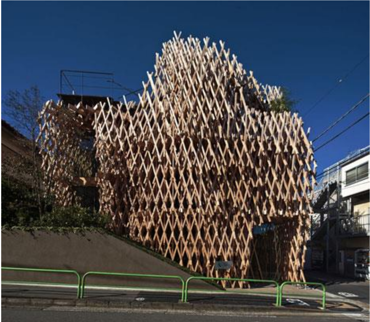
Figure 31. Whilst appearing seemingly complex, the system of interlocking timber members is based on a small number of repeated components. Photo by Daichi Ano
