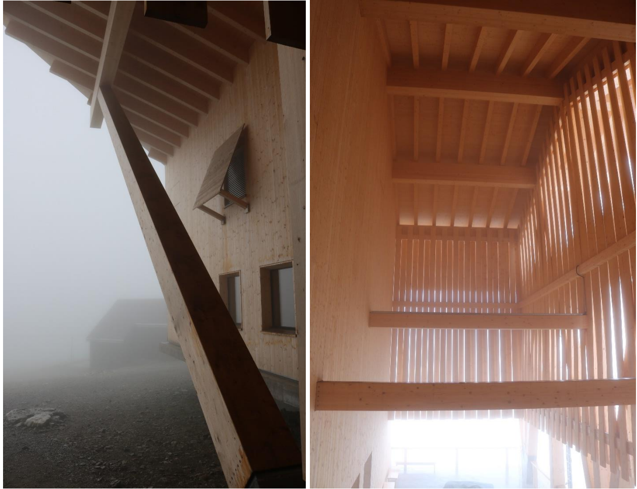
Figure 24 The struts are robust yet appear lightweight from afar. Photos by Author
