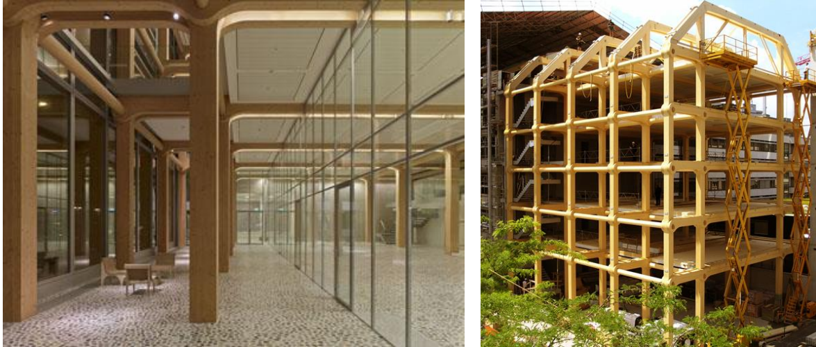
Figure 26 The Circulation along one side of the floor plan allows for a generous void over several storeys, allowing the building to be spatially transparent and to express the timber structure throughout. Photos by Shigeru Ban Architect
