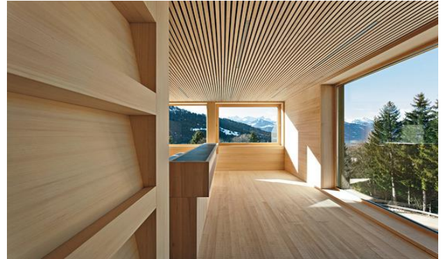
Figure 18 The precise detailing and coordination of the interior CLT panels is evident in the refined interior. Photo by Kucrowicz Nachbaur Architekten
