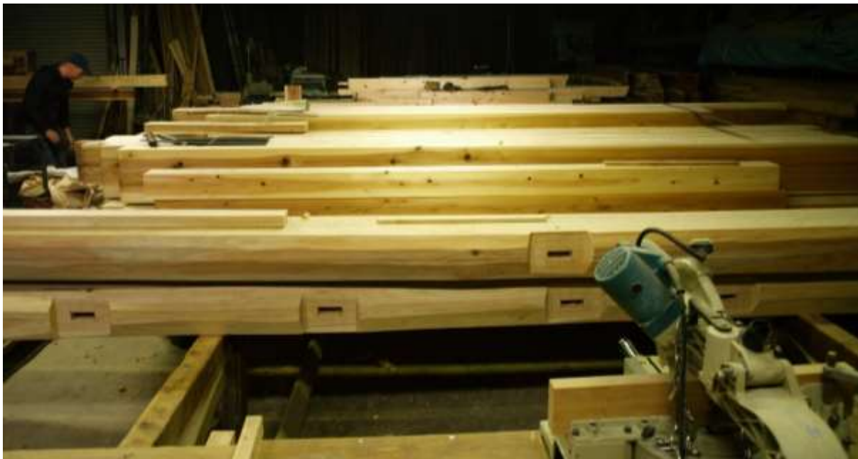
Figure 33 Hand-fabricated frame for a single residence, ready for assembly. Photo: GA
