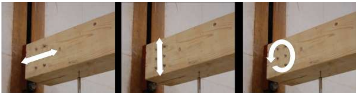
Figure 80 Beam connection doweled slot-in-plate Photo: https://reynoldstom.files.wordpress.com/2013/01/jointmovements.png
