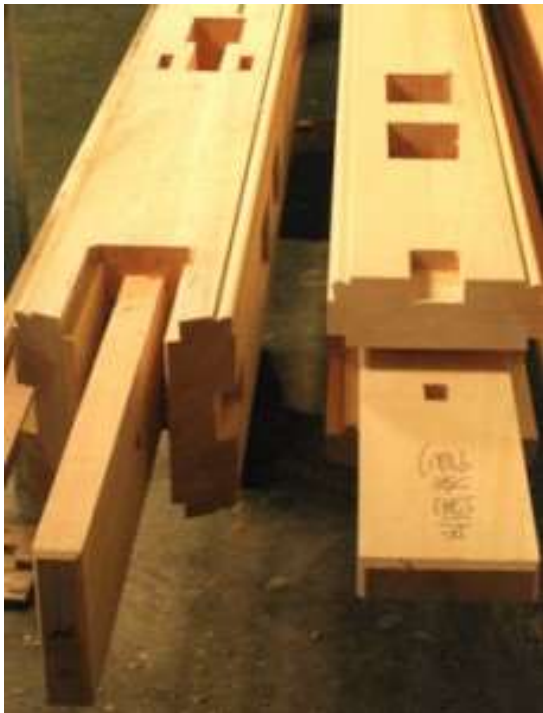
Figure 75 Traditional Post and Beam detail
