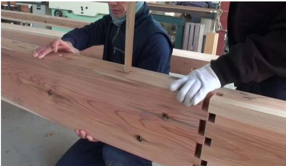
Figure 30 KANAWATSUGI joint during assembly Video: https://youtu.be/W1pvUIQgYtk
