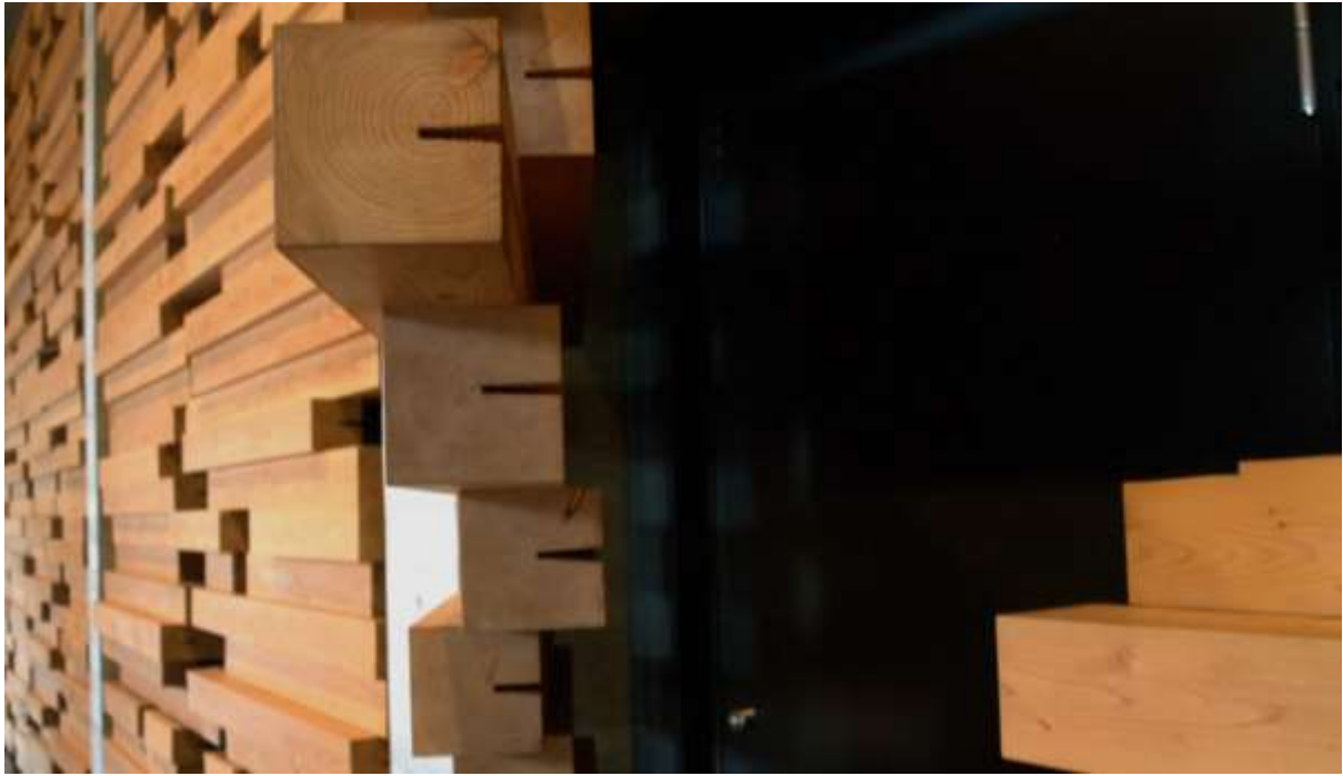
Figure 115 Mokuzaikaikan feature wall. Relief cuts (curfing)to the back of the individual members Photo: GA
