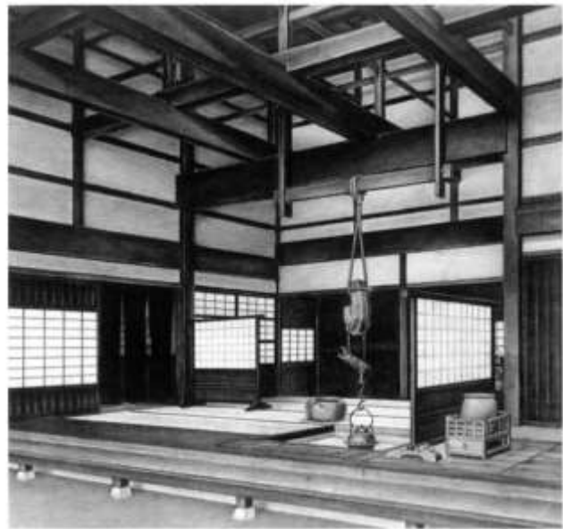
Figure 46 Framing system of Takagi House in Nara (left); Kita House in Ishakawa (right), both early 19th century. [H. Tanahashi & Y. Suzuki Ritsumeikan University, Japan; Embedment Mechanism and Formulation of Major types of traditional wooden joints in Japan ]
