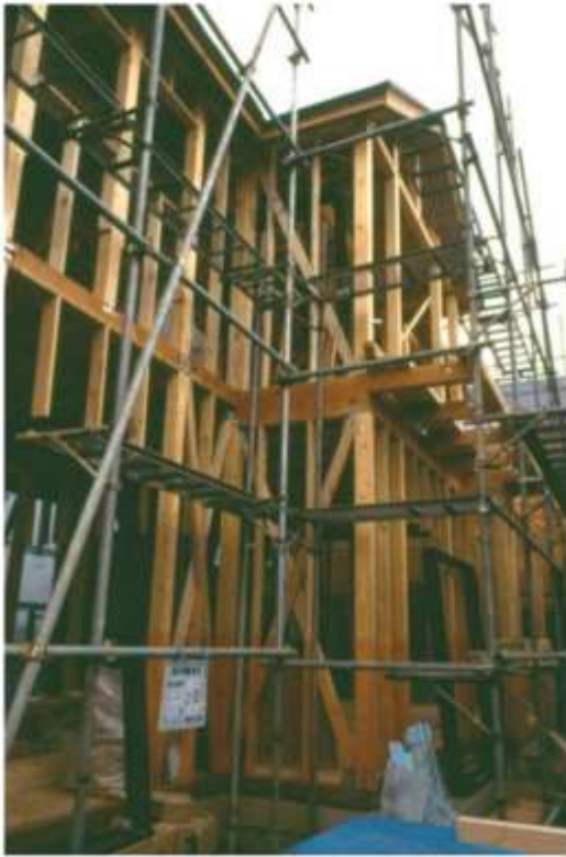
Figure 51 Conventional framing system (post 1950)
