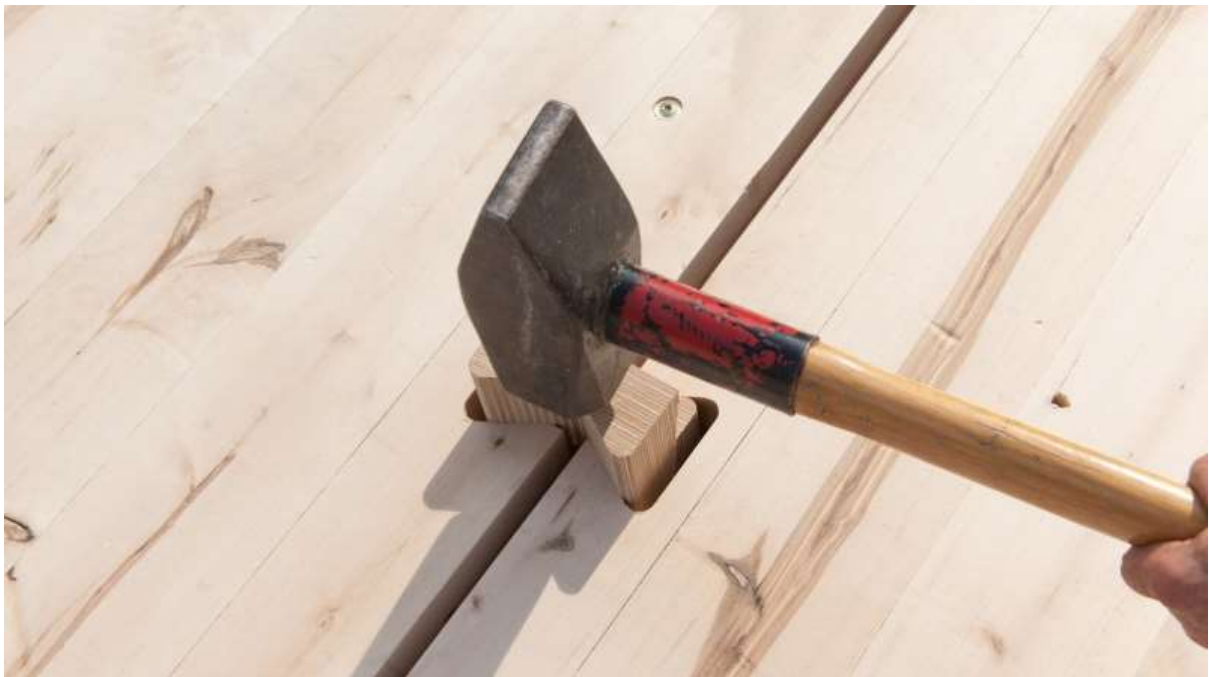
Figure 91 Installation of the X-fix C-type system Phot: http://www.x-fix.at/wp-content/uploads/2016/08/xfix_haus_weichsler_hasslacher023.jpg
