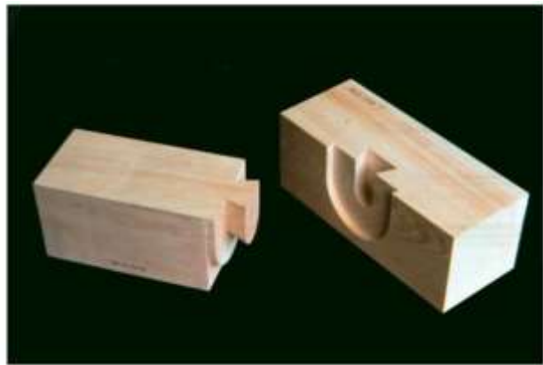
Figure 52 Conventional Post and Beam connection [Mokuzou Kenchiki Kenkyu Forum, Encyclopedia of wood architecture, Gakugei Shuppan, Kyoto, 1995]. (left) Pre-cut joint [Wolfgang Winter] (right)
