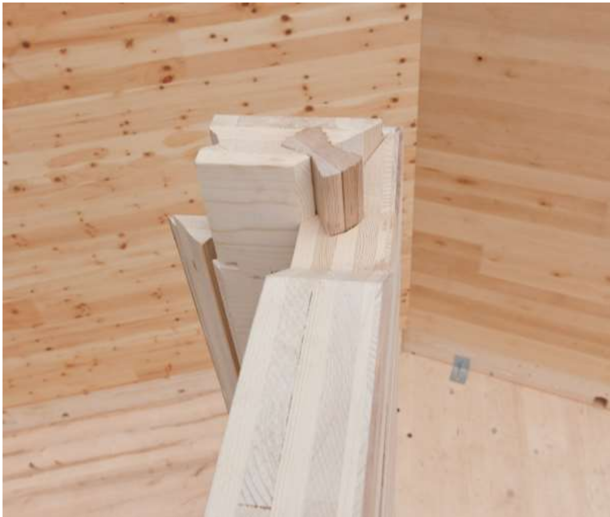
Figure 92 x-fix L-type system Photo: http://www.x-fix.at/wp-content/uploads/2016/08/X-fix-L-eingebaut-hasslacher.jpg
