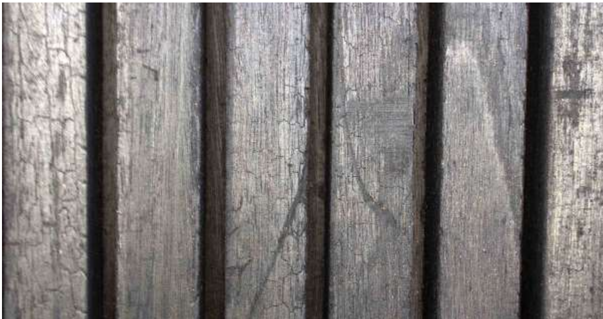
Figure 56 Charred timber profile by ECO TIMBER, Richmond Photo: https://ecotimbergroup.com.au/wp-content/uploads/2017/06/charred_1937.jpg
