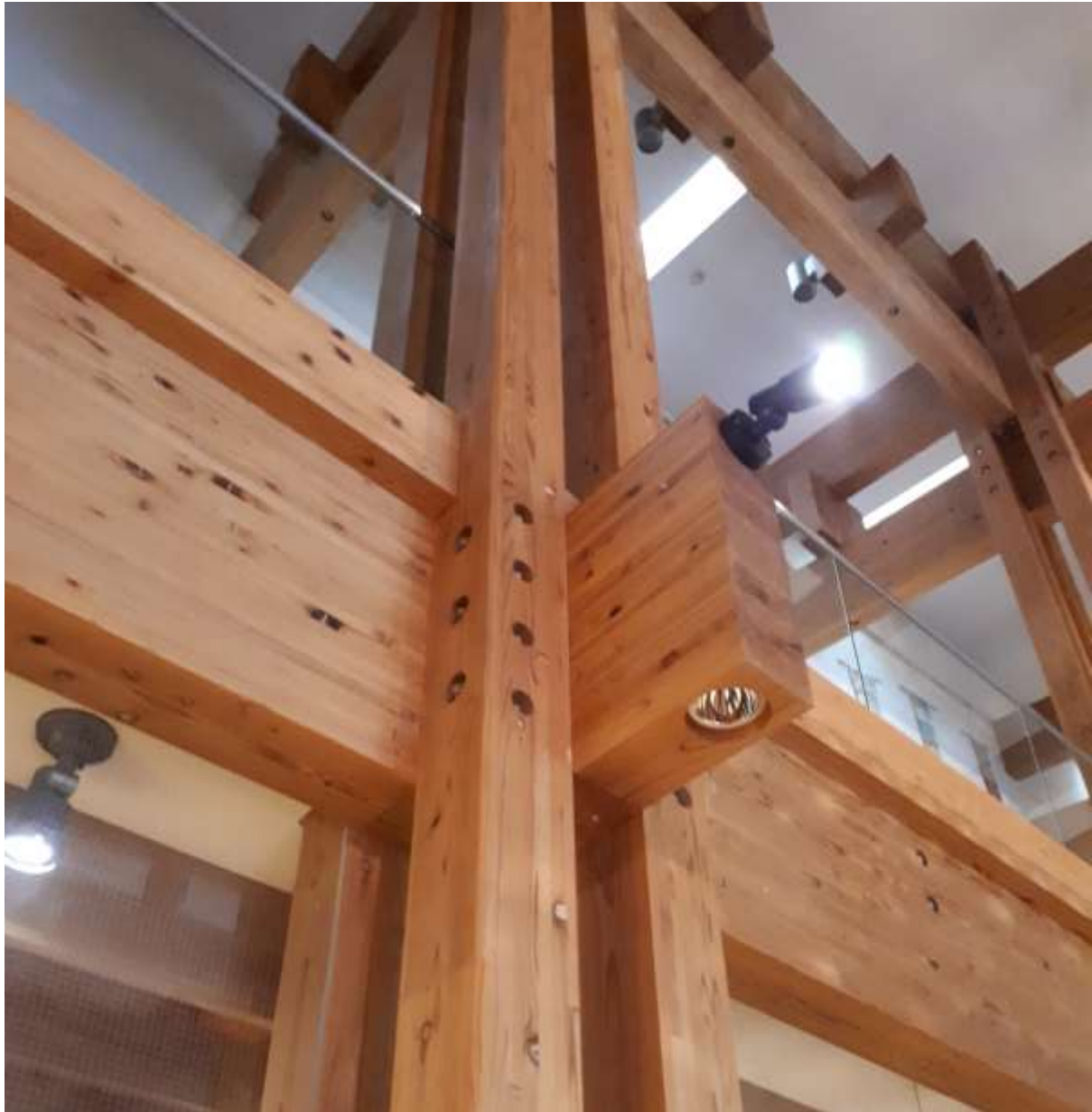
Figure 102 YUSUHARA-CHO column detail. Photo: GA
