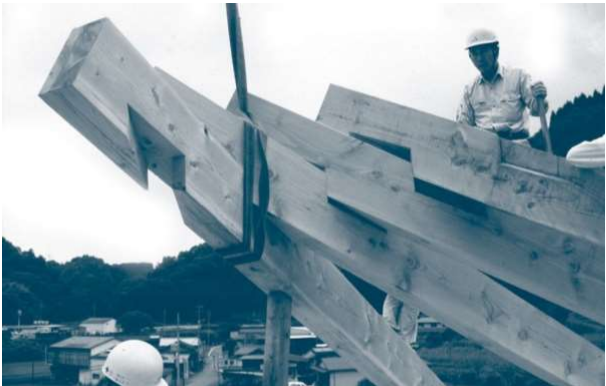
Figure 68 Roof installation of Seiwa Exhibition Hall Photo: https://i.pinimg.com/originals/2f/70/d9/2f70d9d9e5f0651a8b5e6372c9a3b629.jpg
