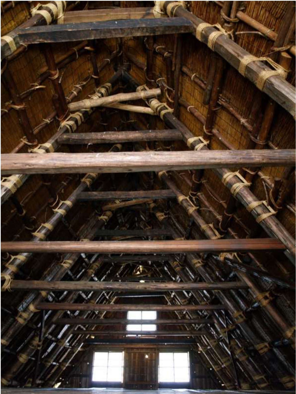
Figure 50 Gasso House Roof in Shirakawa-Go Photo: GA
