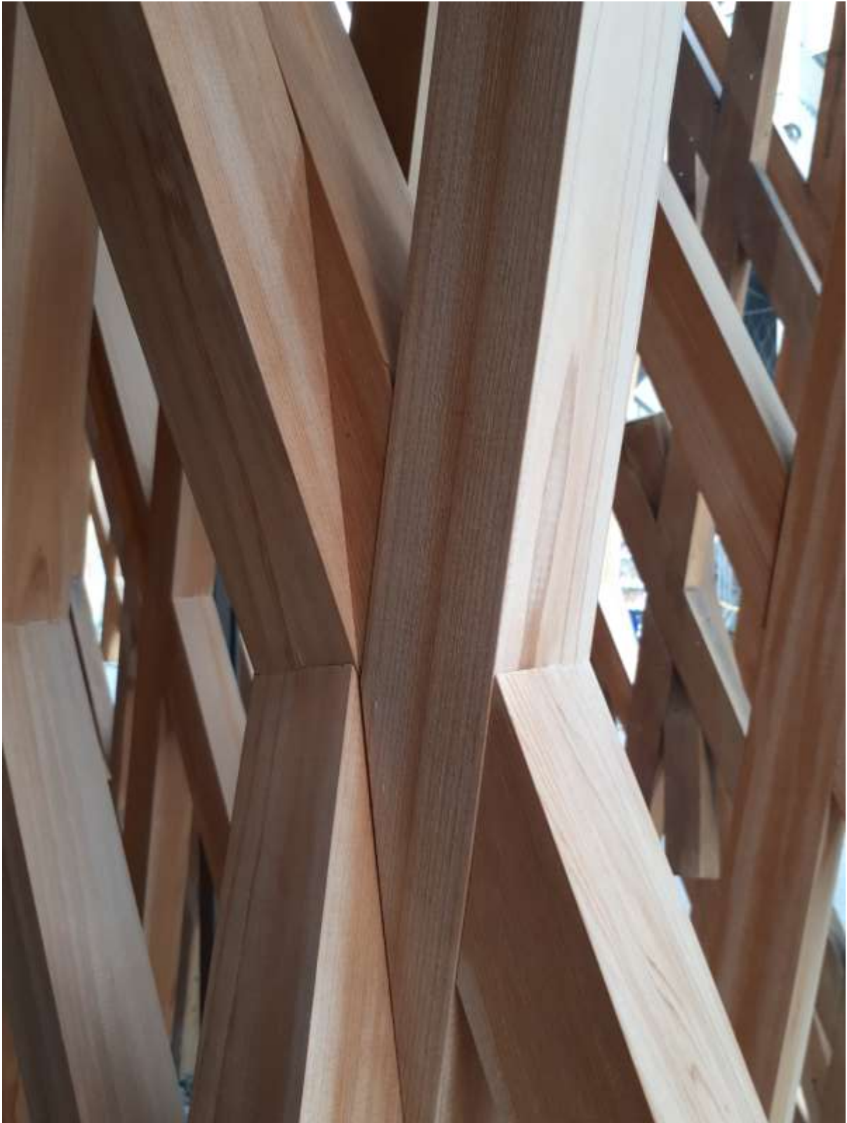
Figure 104 "Hell Set" joint detail. Photo: GA
