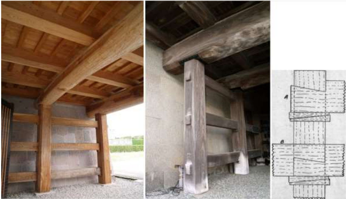
Figure 27 Timber Gates at KANAZAWA Castle; restored (left), original (right) Photo: GA
