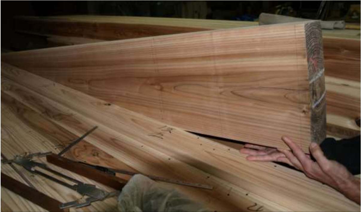
Figure 31 Marked framing members in Zgola's workshop Photo: GA
