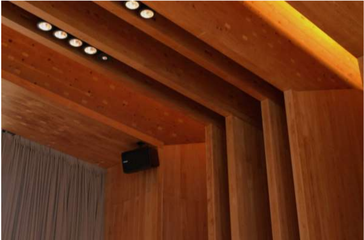
Figure 117 Mokuzaikaikan Composite Beam Detail Photo: GA
